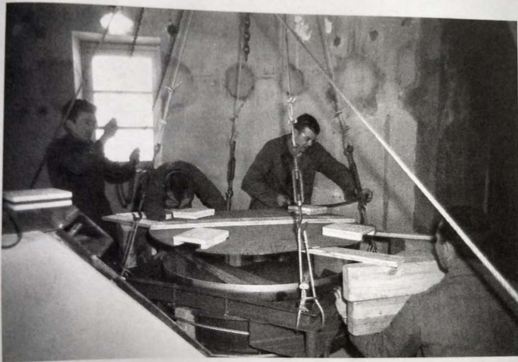
Transporting the one-metre mirror in the telescope tower in March 1962
